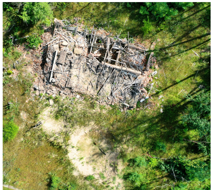
Aerial view taken by a drone showcasing a destroyed building during non-technical survey (July 2023).
